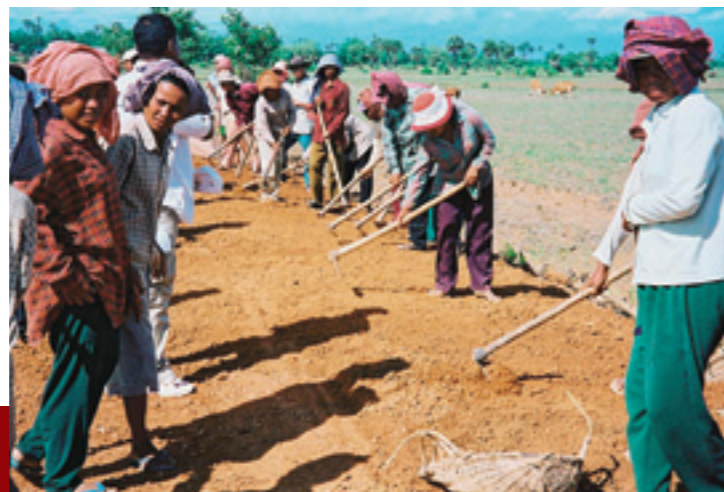
A joint effort: rural road construction
